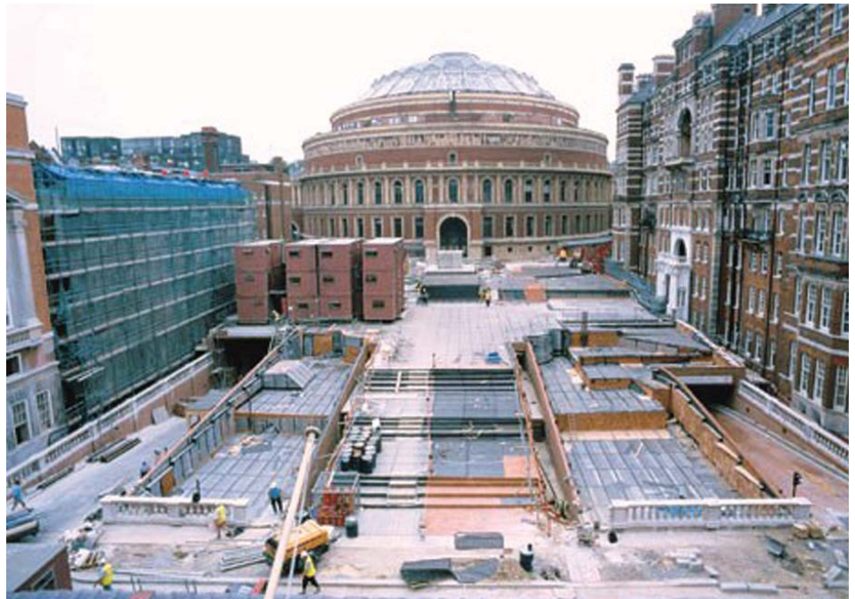
Waterproofing around the Albert Hall
